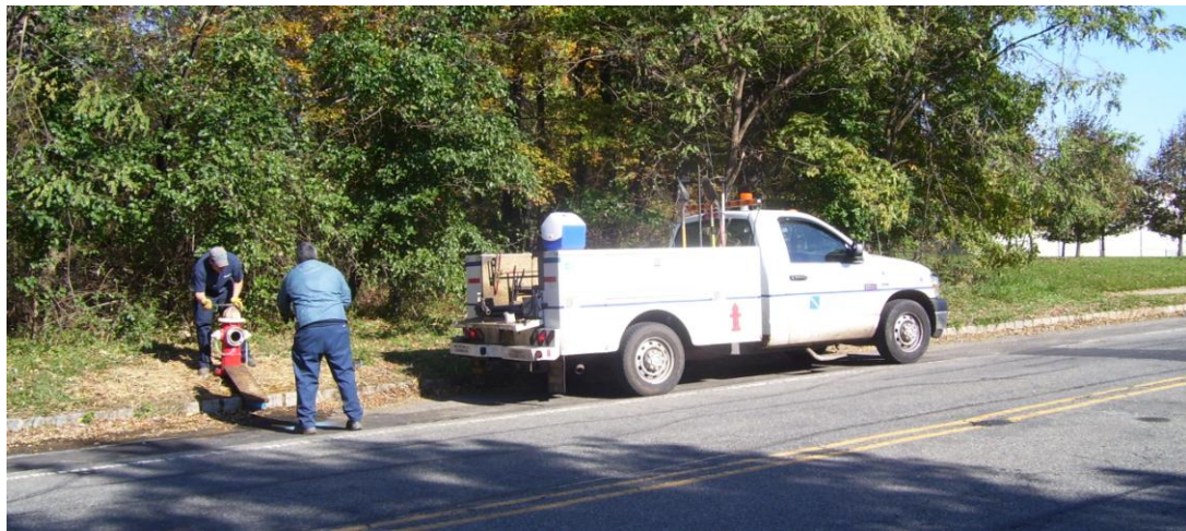
Crews from Southeast Morris County Water District service hydrant on Eden Lane.
